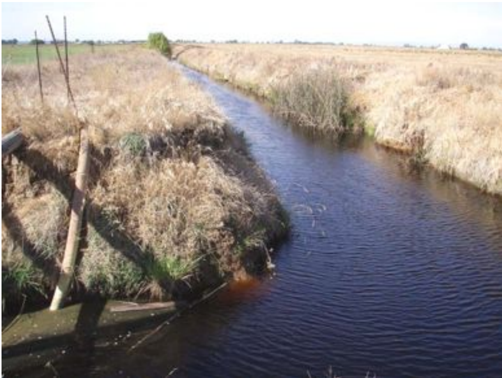
C-Promenade looking downstream
