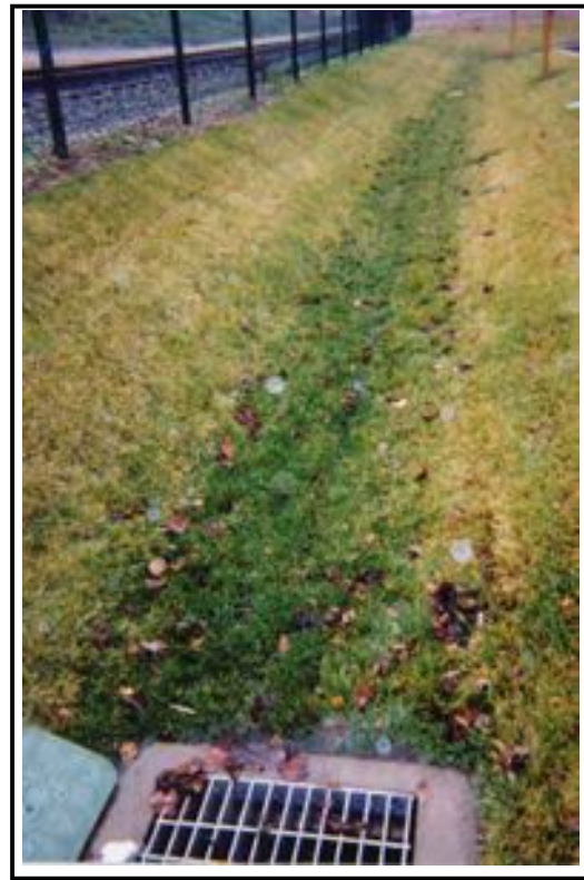
Figure 3. Photograph of the RAS vegetated swale during a sampling event.
