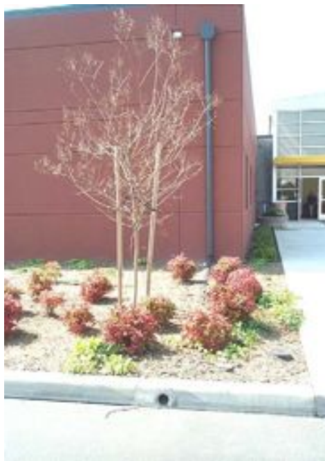
Figure 4. Photograph of a downspout from the RAS facility. Sampled aliquots were collected at the outlet in the curb.
