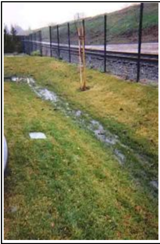
Figure 3. Photograph of the RAS vegetated swale during a sampling event.
