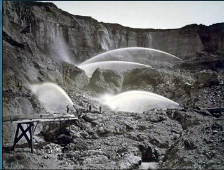
Hydraulic monitors in operation, North Bloomfield mine, circa 1880s, Malakoff Diggings, Nevada County
