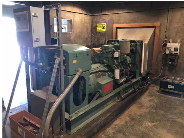
Figure 5: Emergency Electric Generator
