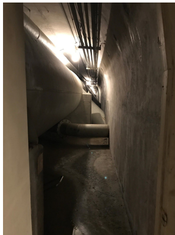
Figure 6: Underground Pipe Connecting Reservoir to the North Fork of Cache Creek
